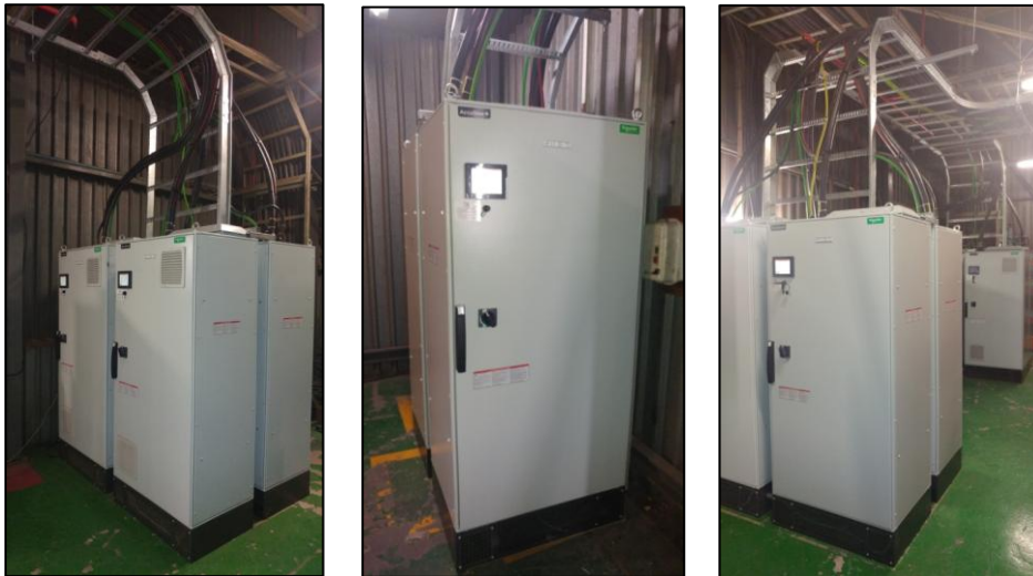
Figure 2: AccuSine PCS+ AHF Units in Paintshop Substation
